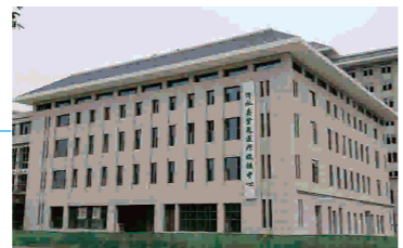
工程名称: 甘肃天水清水县医疗救援中心 主机类型: GSG系列 Project name: Qingshui county Medical rescue center GSG series Ground Source HP screw chiller
