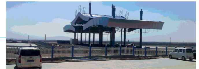
工程名称: 山西河津吉河高速河津北服务区 主机类型: GSG系列 Project name: Jihe highway service station GSG series Ground Source HP screw chiller 建筑面积: 6,000m 2 装机容量: 1080kw Covered area: 6,000m 2 Capacity: 1080kw
