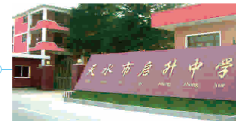
工程名称: 甘肃天水启升中学 主机类型: GSG系列 Project name: QI SHENG High School, Tianshui GSG series Ground Source HP screw chiller
