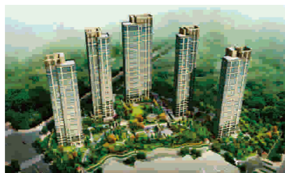
工程名称: 山东青岛上实上海 主机类型: GSG系列 Project name: Shanghai shandong Qingdao. On the sea GSG series Ground Source HP screw chiller
