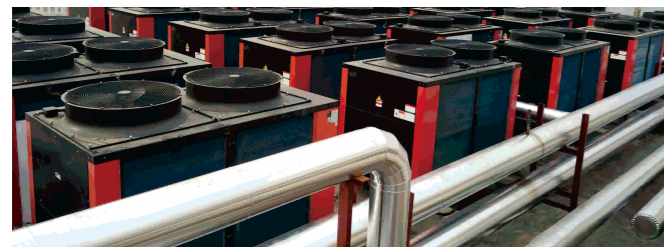
工程名称: 山东淄博寨里镇热泵改造 主机类型: WACM系列 Project name: Renovation of the heat pump in Zhaili town WACM series Air cooled modular chiller 建筑面积: 341,000m 2 装机容量: 13640kw Covered area: 341,000 m 2 Capacity: 13640kw
