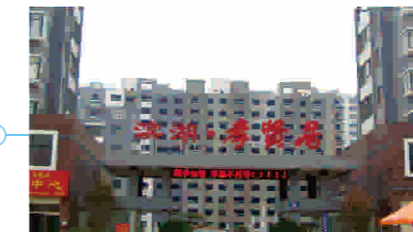
工程名称: 山东济宁滨湖孝贤居小区 主机类型: GSG系列 Project name: Binghu housing district GSG series Ground Source HP screw chiller
