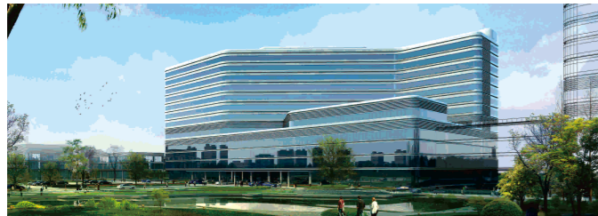
工程名称: 浙江宁波妇女儿童医院北部院区 建筑面积: 138,000m 2 主机类型: GSG系列 Project name: Women's and Children's Hospital GSG series Ground Source HP screw chiller Covered area: 138,000m 2 Capacity: 6100kw
